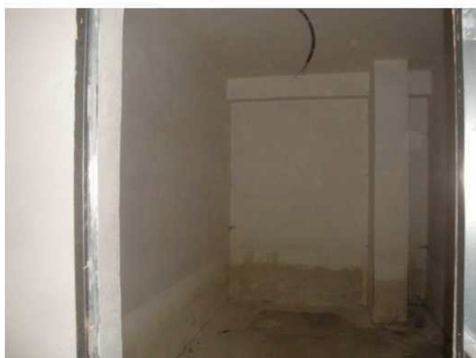
Cantinola piano interrato
