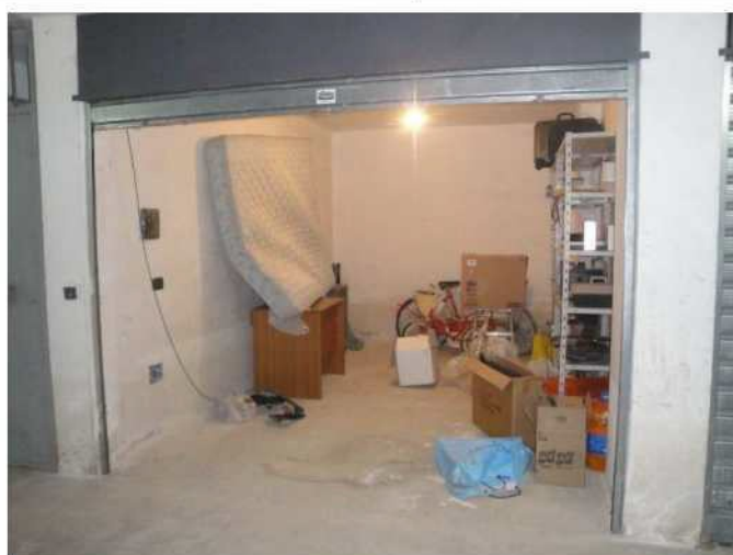
Box piano interrato
