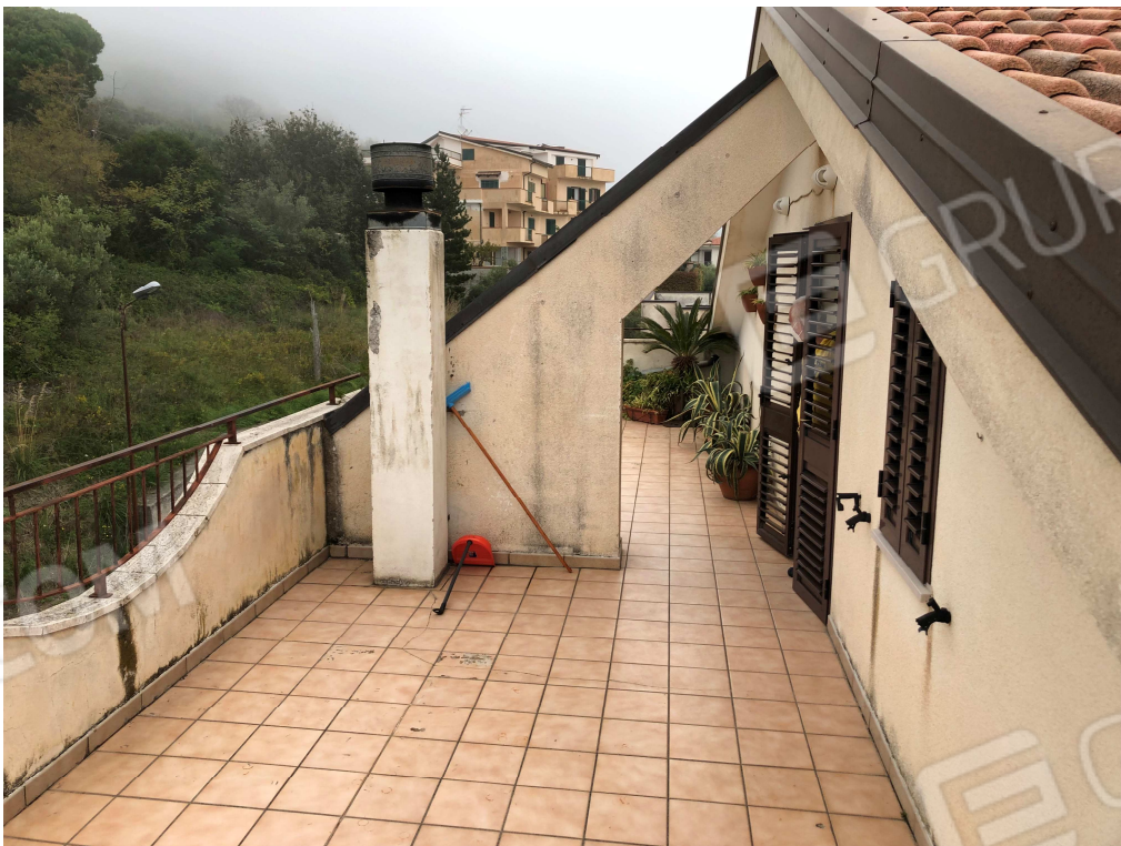
Terrazzo al piano mansarda
